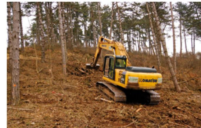
Clearing of tree crown cuttings and uprooting of rootstocks using an excavator
